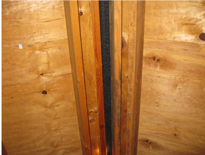
Photo 1 – current ridge vent
